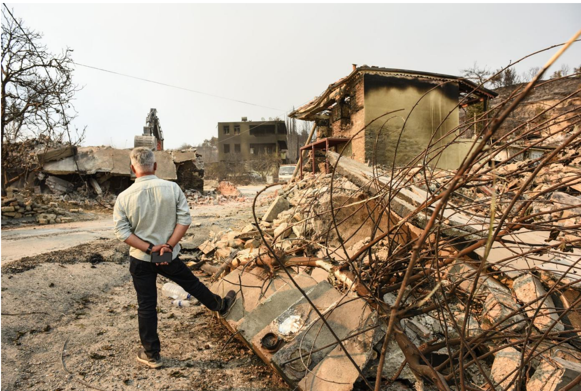
A resident in Kalemler stands next to the rubble of a neighbour’s house and looks at the burnt remains of his own home (MEE/Yusuf Selman Inanc)
