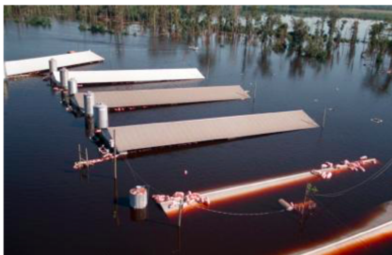
Submerged CAFO confinement buildings containing thousands of trapped, drowned and eventually rotting pigs that could not be rescued
