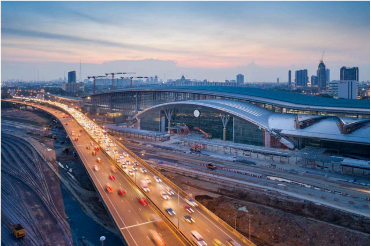
Thailand's massive Bang Sue Grand Station nears completion and will serve as a terminal for Chinese-built high-speed trains.
