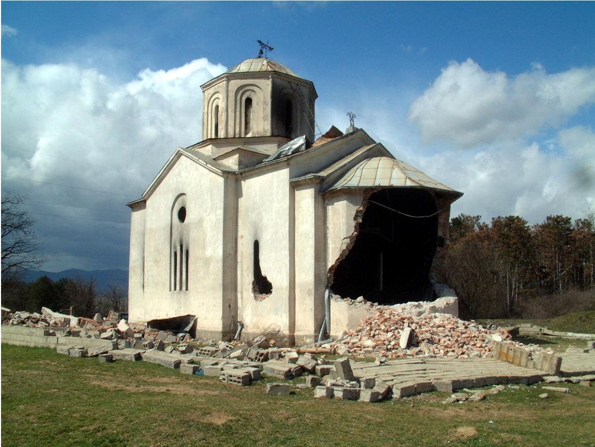
Serbian Orthodox church of St. Elijah in Podujevo destroyed in 2004 unrest by Kosovo Albanians (Licensed under CC BY 2.0)
