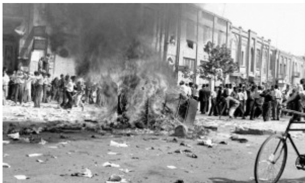
Newspaper office burned in Tehran during 1953 US coup in Iran.
