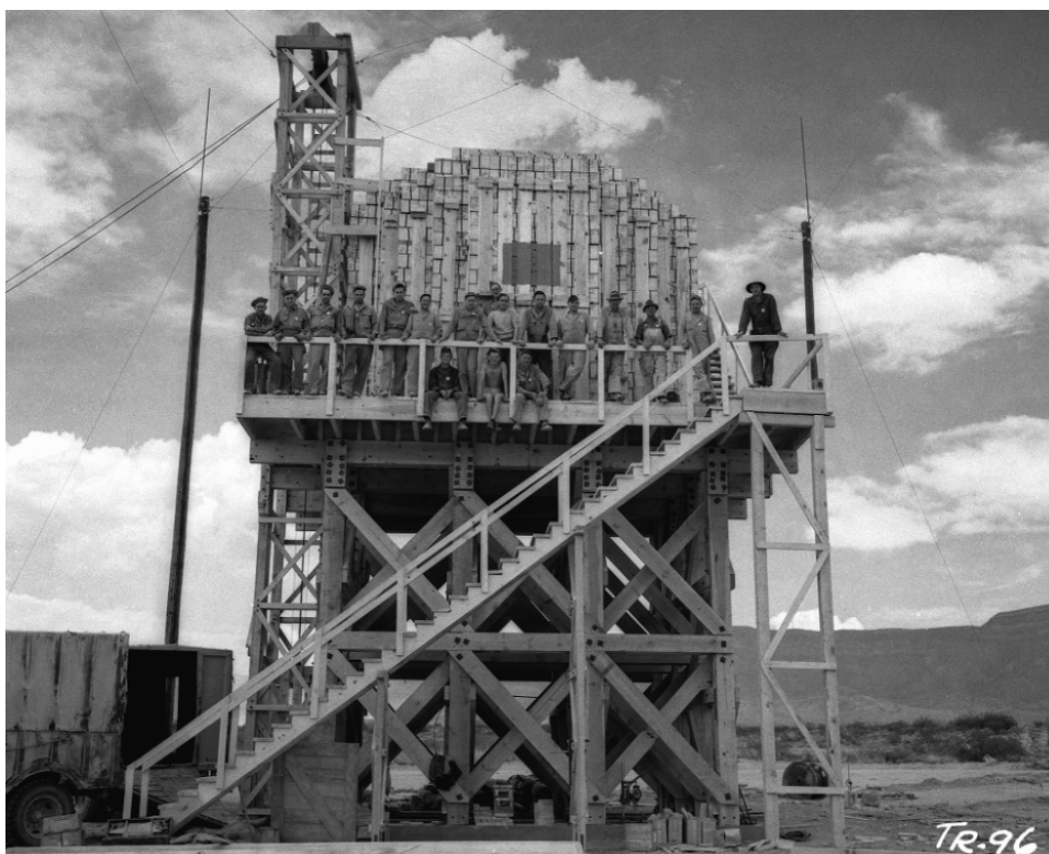
Figure 3. The Trinity project was actually two “shots,” one non-nuclear, and one-nuclear. The first test, on May 7, 1945, was of conventional explosives, designed to help calibrate the instruments before the atomic test. This device was threaded with 1,000 curies of radioactive materials produced in the Hanford reactor, so that the dispersal of radioactivity could be studied. Here the test crew stands triumphantly with 108 tons of TNT in the background. Image courtesy of Los Alamos National Laboratory’s National Security Research Center library.
