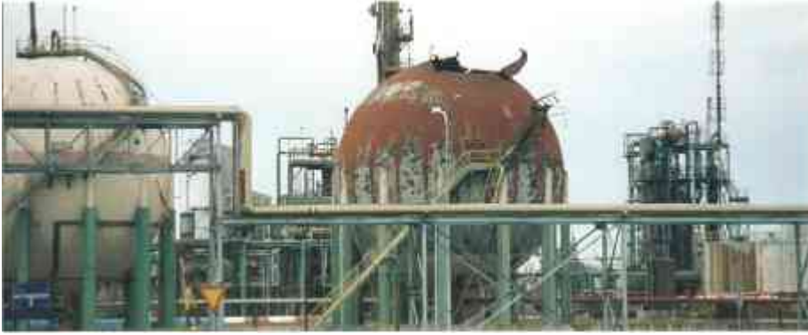
Pancevo Chemical Plant bombed by NATO. M. Chossudovsky, 2000
