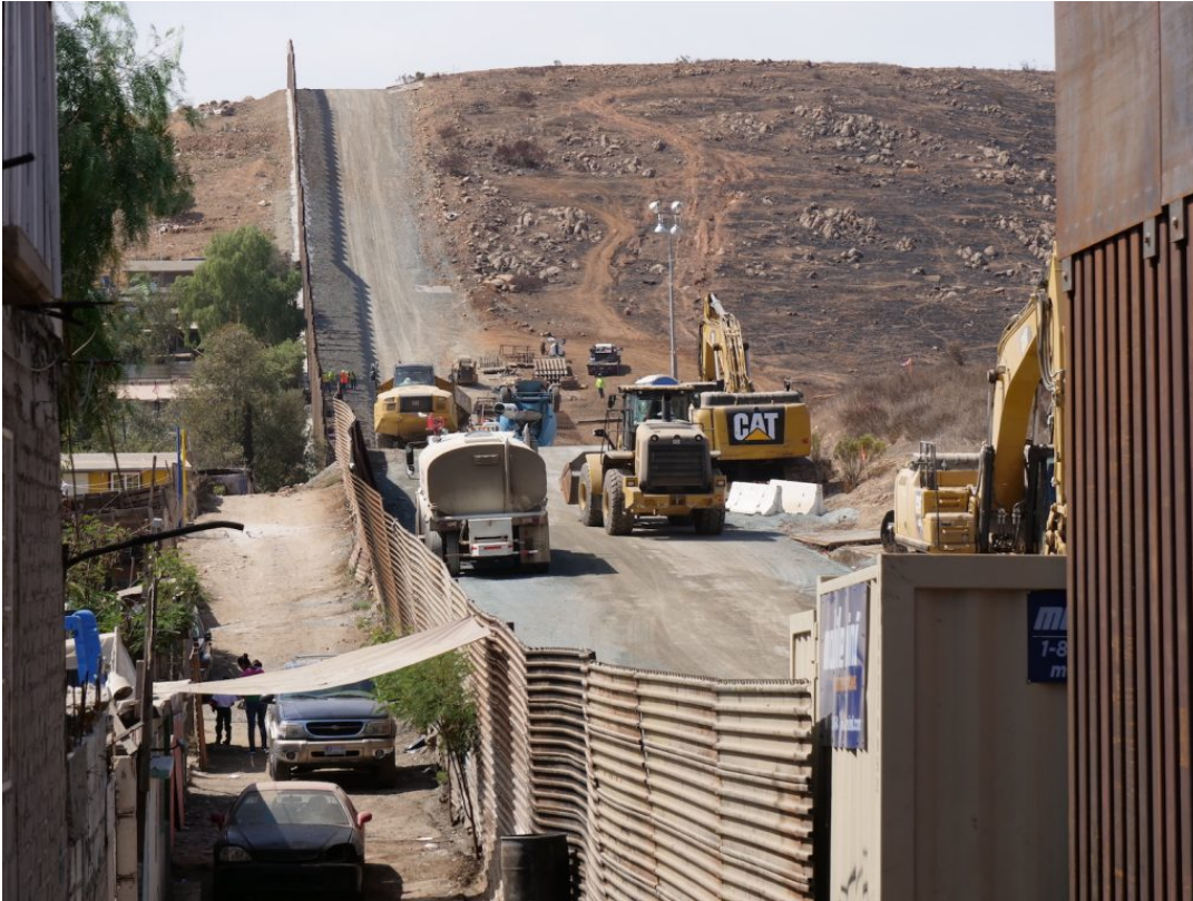
Construction of US-Mexico wall
