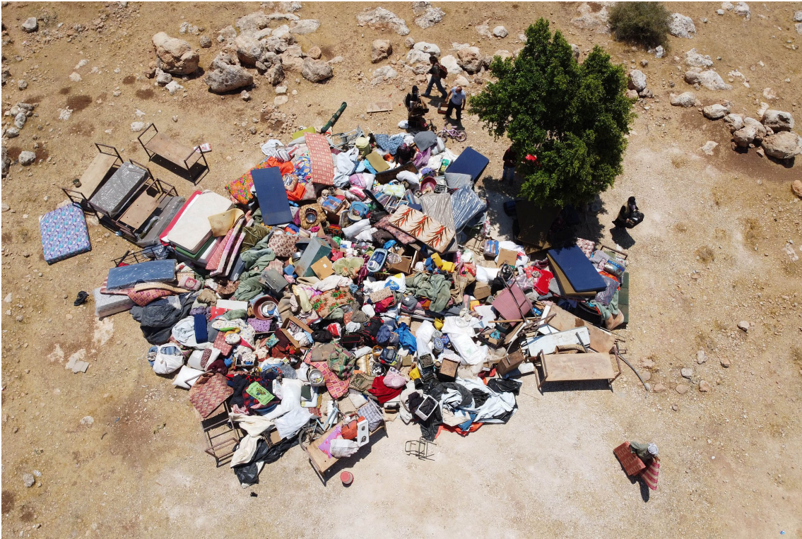
An aerial photo of the demolition of the Khirbet Humsa community in the Jordan Valley, occupied West Bank, July 8, 2021. (Oren Ziv)
