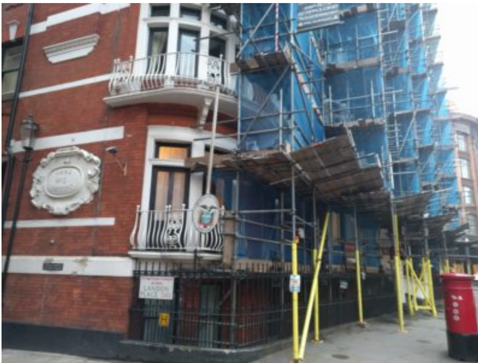
Scaffolding near balcony where Assange has appeared. (Sean O'Brien)
