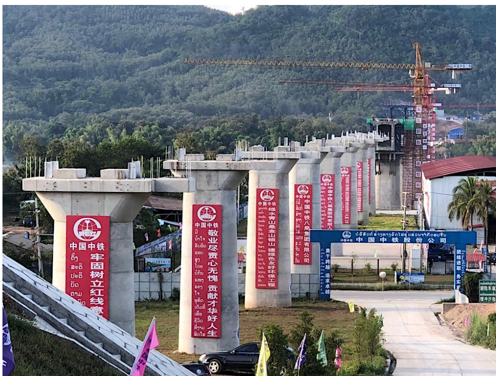
Laos - BRI project. China building high-speed train
