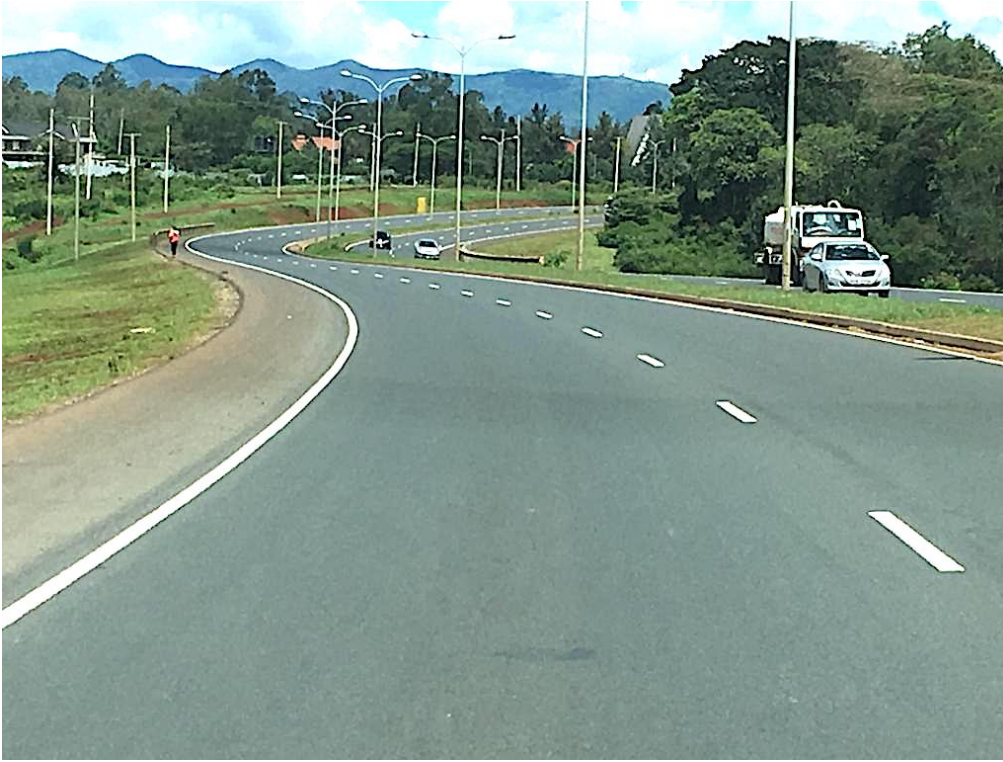
Africa - BRI. New China-built highway
