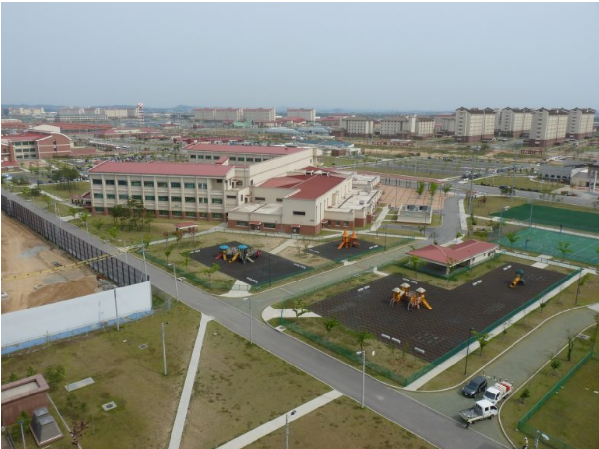
Newly built soldier housing, schools and other facilities as seen from the balcony of a 12-story residential tower. In 2006, the South Korean government forcibly relocated Korean farming villages in order to expand what will be America's largest overseas military base. Photo by Jon Letman.
