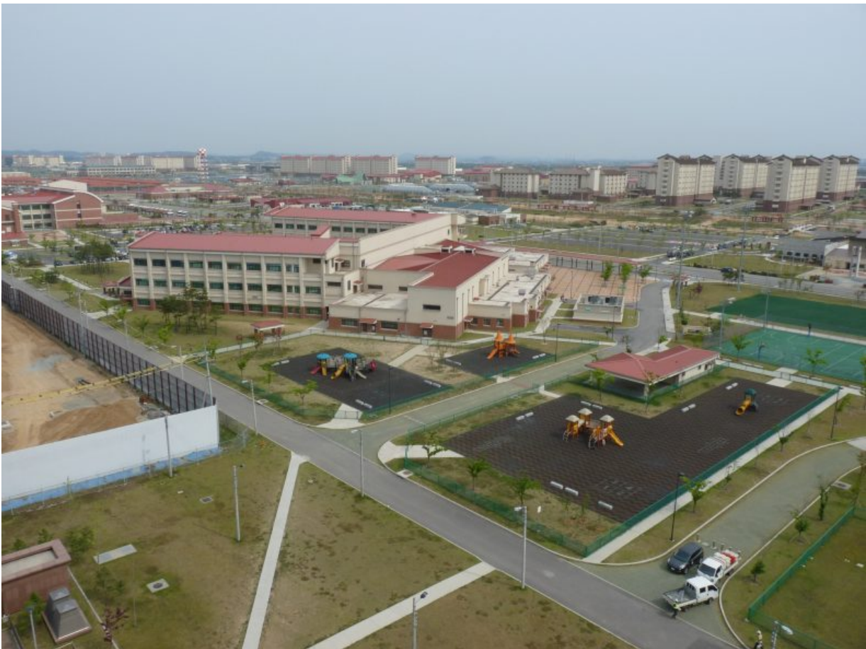
Newly built soldier housing, schools and other facilities as seen from the balcony of a 12-story residential tower. In 2006, the South Korean government forcibly relocated Korean farming villages in order to expand what will be America's largest overseas military base. Photo by Jon Letman.
