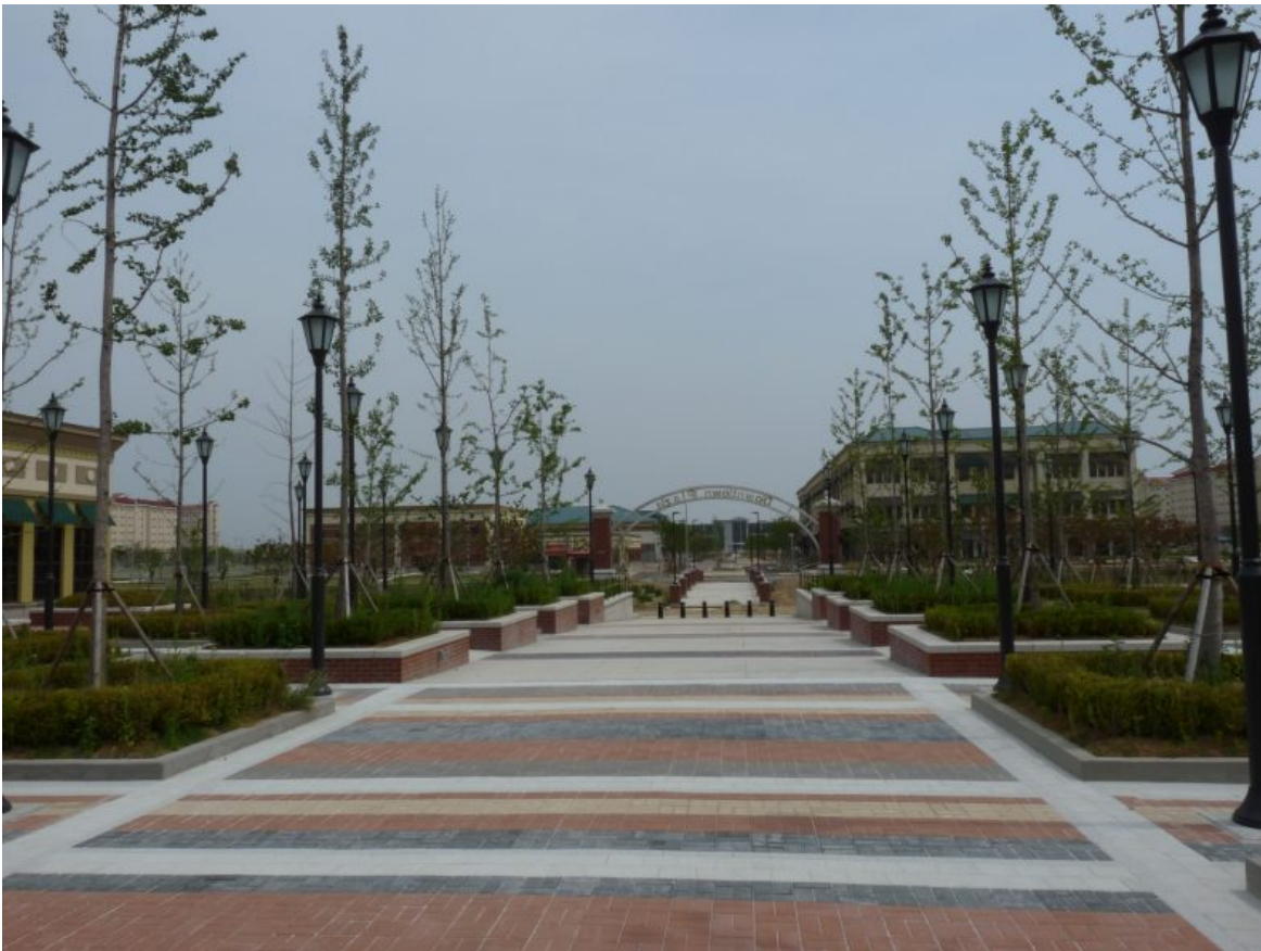
Part of the U.S. military’s largest overseas base includes this newly-built pedestrian-friendly downtown plaza. The 3,454 acre installation will eventually be home to around 45,000 military personnel, their
