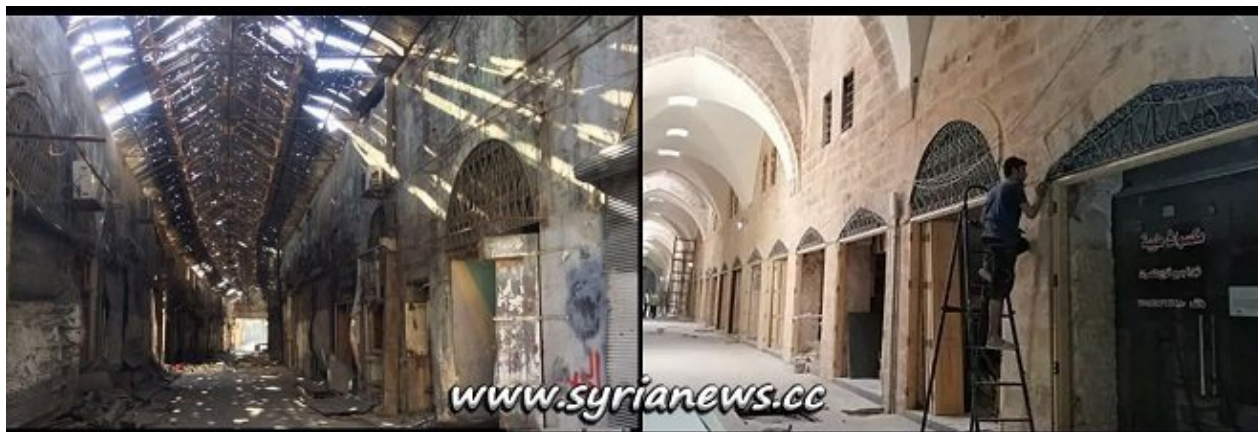
Rebuilding Aleppo Bazaar
