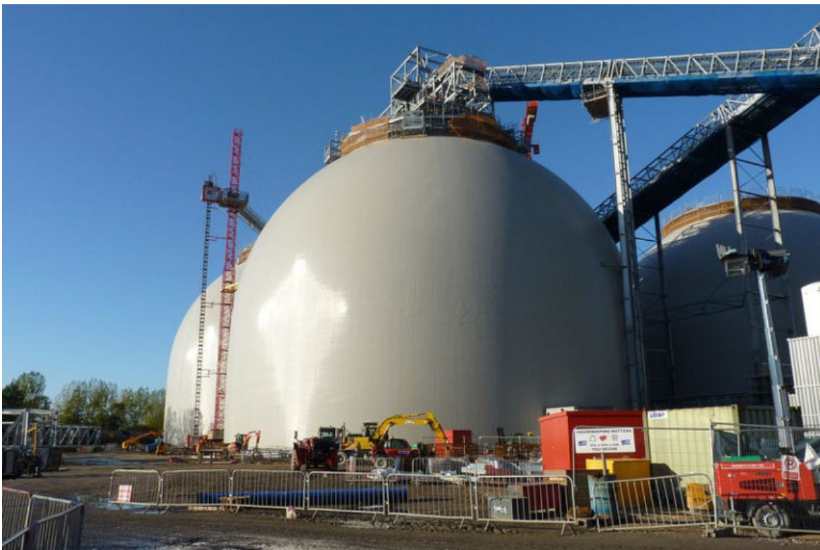
The Drax power station in the UK, one of the world’s largest users of woody biomass to make energy. The uncounted carbon from wood pellets burned at Drax flows into the atmosphere, adding to climate change. Photo credit: DECCgovuk on VisualHunt / CC BY-ND.
